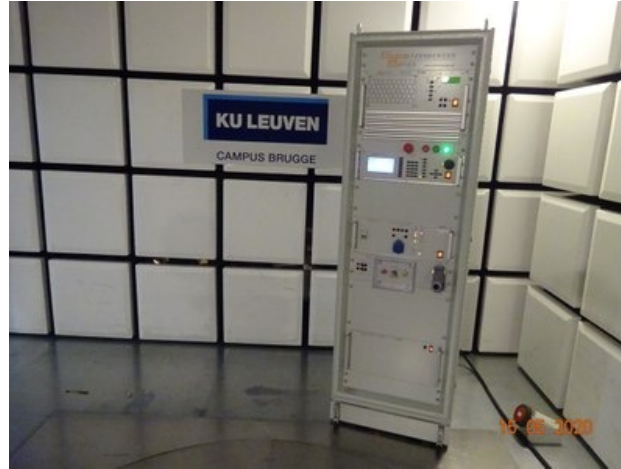
High-end Power analysis system for harmonic emission and Flicker
